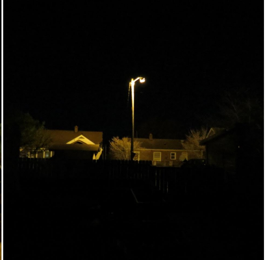
Shield blocks light trespass
