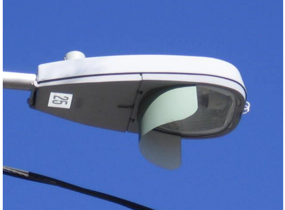
Shield orientation is adjustable
