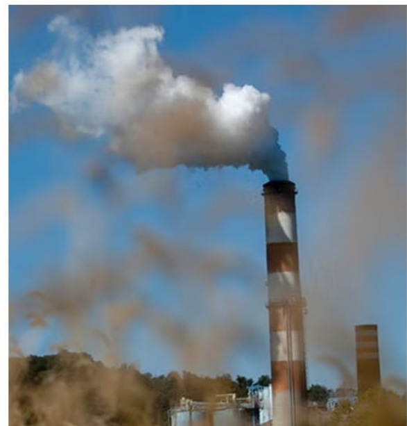
A power plant in New Eagle, Pa.. (Jeff Swensen/Getty Images)
