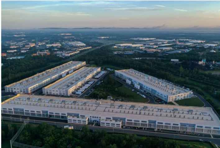
An Amazon Web Services data center in Manassas, Va. PHOTO: NATHAN HOWARD/BLOOMBERG NEWS
